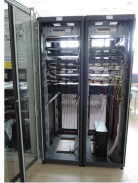
Figure 5: Core components of the public access Wi-Fi network are hosted in a rack at the control centre.
